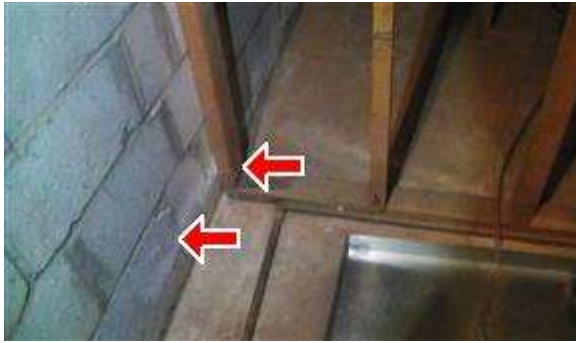
13.3 Picture 10. Efflorescence
