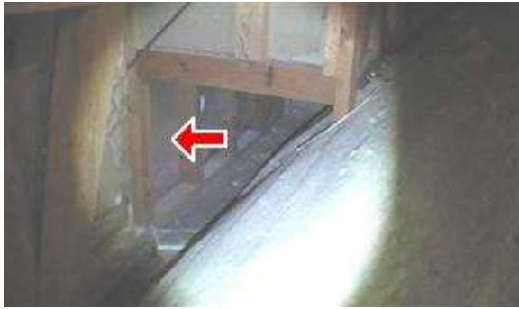
13.2 Picture 3 missing insulation
