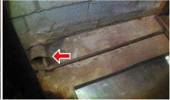
13.3 Picture 11. Drain with moisture signs
