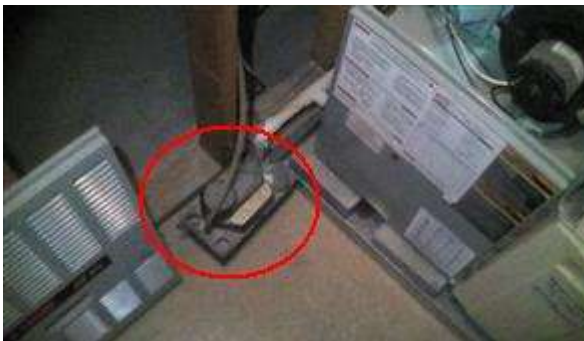
8.2 Picture 3. Place into a drip pan
