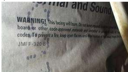
13.2 Picture 1. exposed paper is a fire hazard
