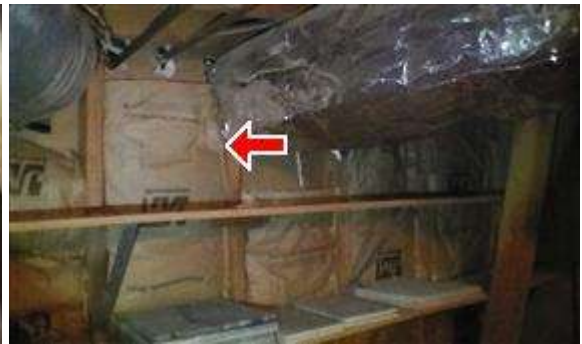
13.2 Picture 1. exposed paper is a fire hazard
