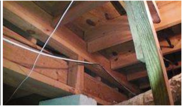
13.2 Picture 4 Need insulation under the floor
