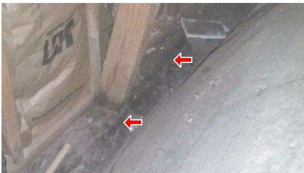
13.4 Picture 3 water intrusion area
