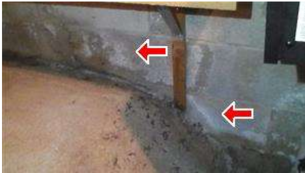
13.3 Picture 14 Efflorescence
