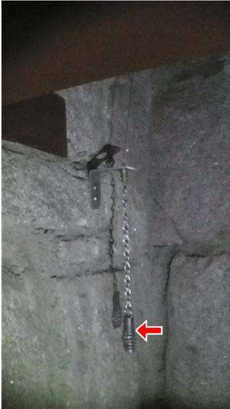
15.1 Picture 4. Current damper control
