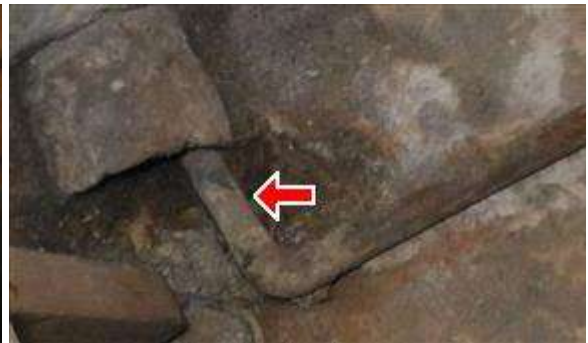
13.3 Picture 13. T&P drain line termination
