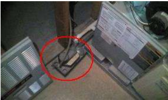
8.2 Picture 3. Place into a drip pan
