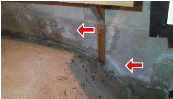
13.3 Picture 14 Efflorescence
