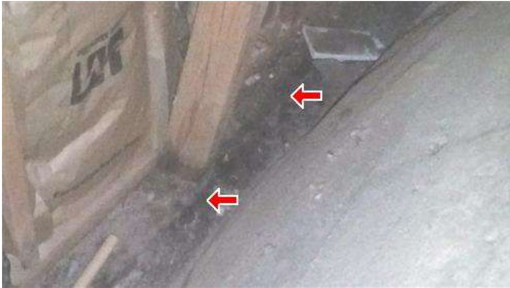
13.4 Picture 3 water intrusion area
