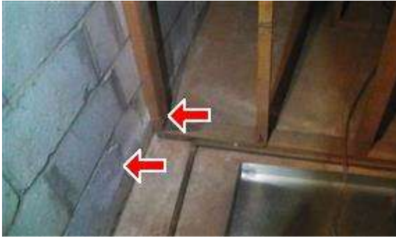
13.3 Picture 10. Efflorescence
