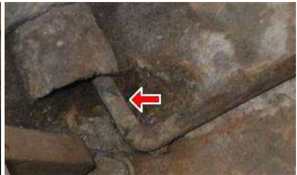
13.3 Picture 13. T&P drain line termination
