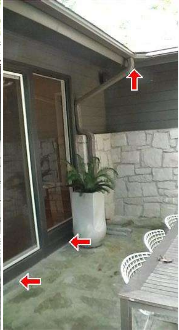
13.3 Picture 9. Water collection area brings water into the crawl
