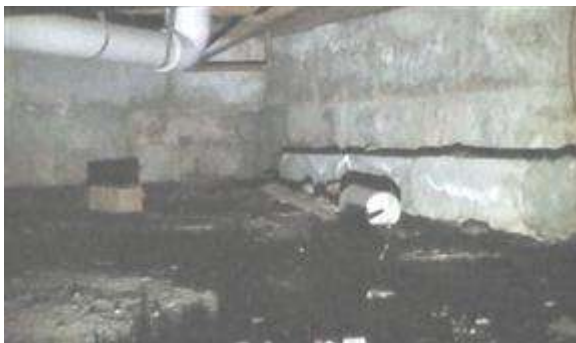
13.3 Picture 17. Entry point for water
