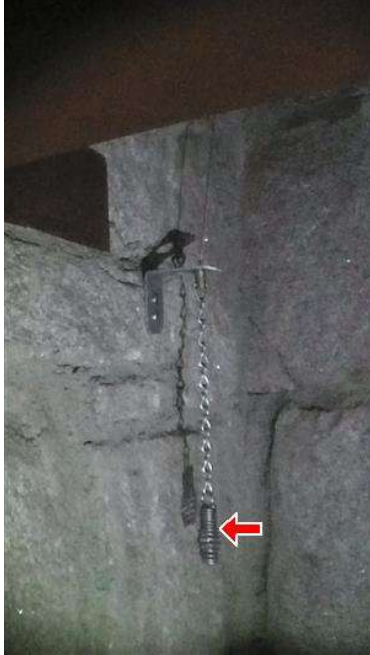
15.1 Picture 4. Current damper control
