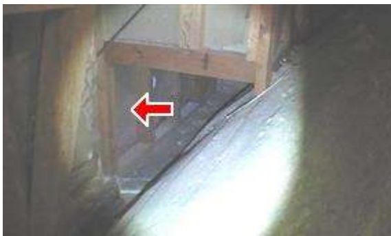
13.2 Picture 3 missing insulation
