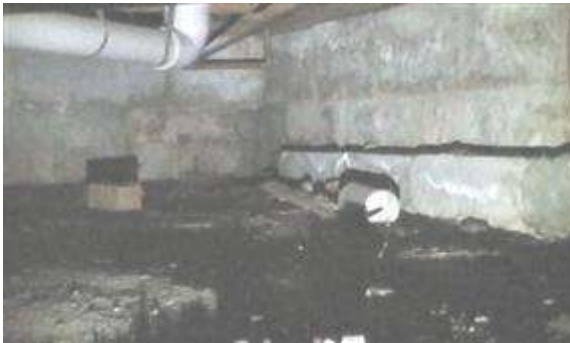
13.3 Picture 17. Entry point for water
