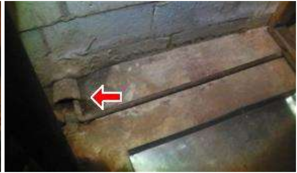
13.3 Picture 11. Drain with moisture signs
