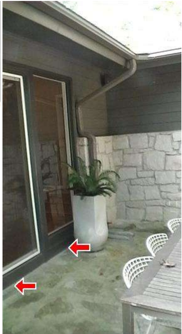
13.3 Picture 7. Exterior patio is higher than the top of the foundation wall
