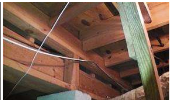
13.2 Picture 4 Need insulation under the floor
