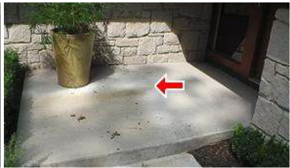
3.5 Picture 2. Water currently spills over the valley at the front entrance
